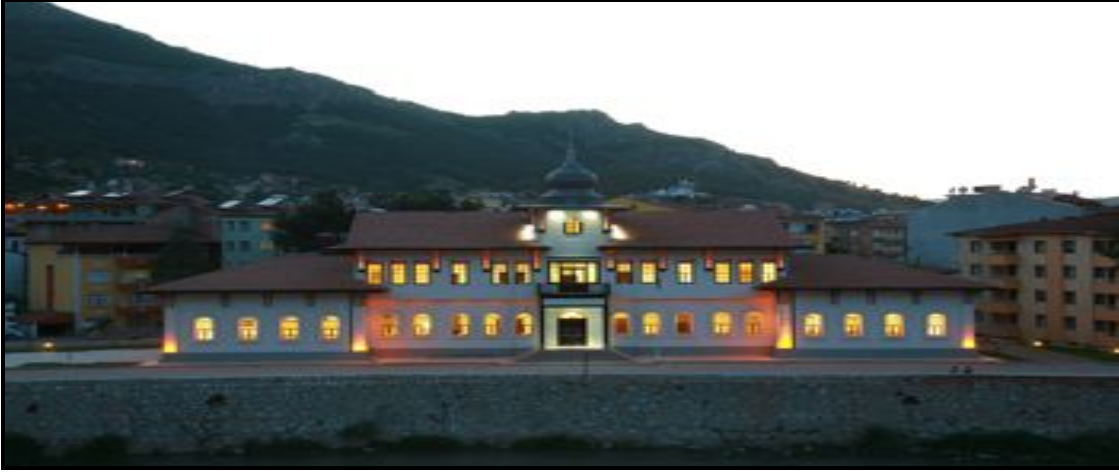
Figure 3.10.7.1.5 Milli Mücadele Museum and Convention Centre, Source:( http://www.amasyakulturturizm.gov.tr ), ( http://amasya05.wordpress.com ), Amasya Province Strategic Plan 2007-2011
