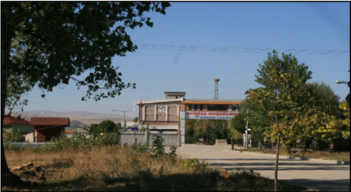
Figure 3.10.5.3 Gözlek Thermal Facilities
